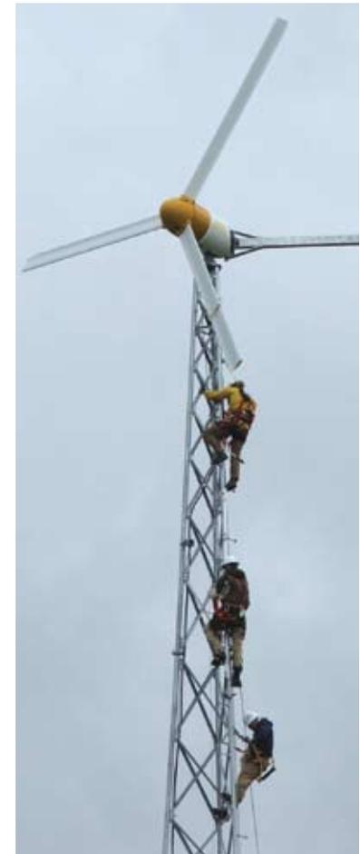
Buckeye Power and Logan County Electric Cooperative installed a demonstration 10-kilowatt wind turbine at Indian Lake High School in 2006.
